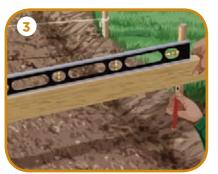
Establish the finish grade and slope or pitch of pavement to allow for drainage. Lay out the lines and corners with string line and stakes. Compact sub-base with mechanical compactor.
