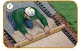
Spread 1" of concrete sand evenly over the compacted base. Screed the bedding sand to a level, smooth surface using a screed board. For areas wider than the width of the screed board, use 1" conduit pipe as screed guides 4' apart. Screed sand, remove screed rails & fill in depressions with fresh sand. You should end up with a complete layer of smooth sand. Do not disturb sand bed after it has been screeded.
